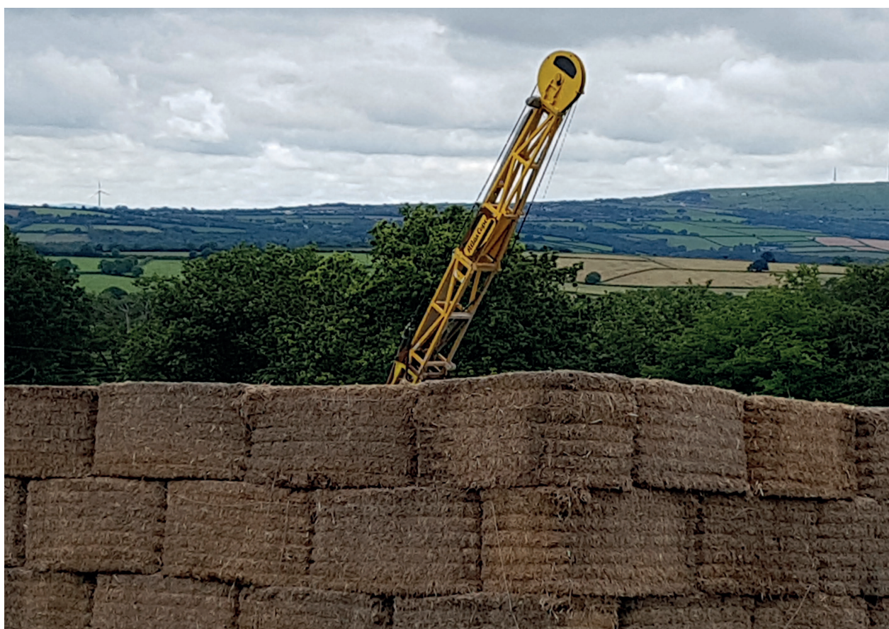
Figure 17: Breaking down barriers for responsible sourcing of critical minerals. Exploration for critical minerals in South West England uses hay bales for both noise attenuation and to reduce visual impacts of drilling, in sensitive areas. Hay bales are not always required, each drill site needs to be assessed following noise surveys and site inspections, as well as discussions with the community. Source: Cornwall Resources Ltd
