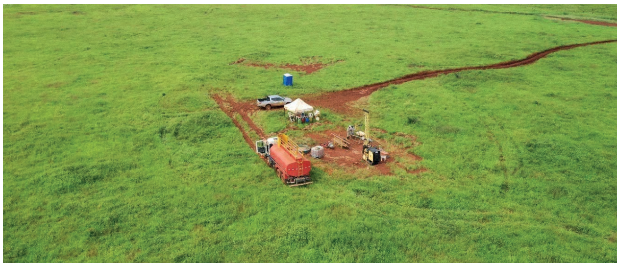
Project site in March 2022.
